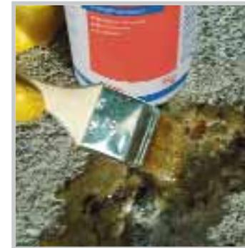
Apply the mortar directly into the fresh primer, trowel off and smooth to finished level...
